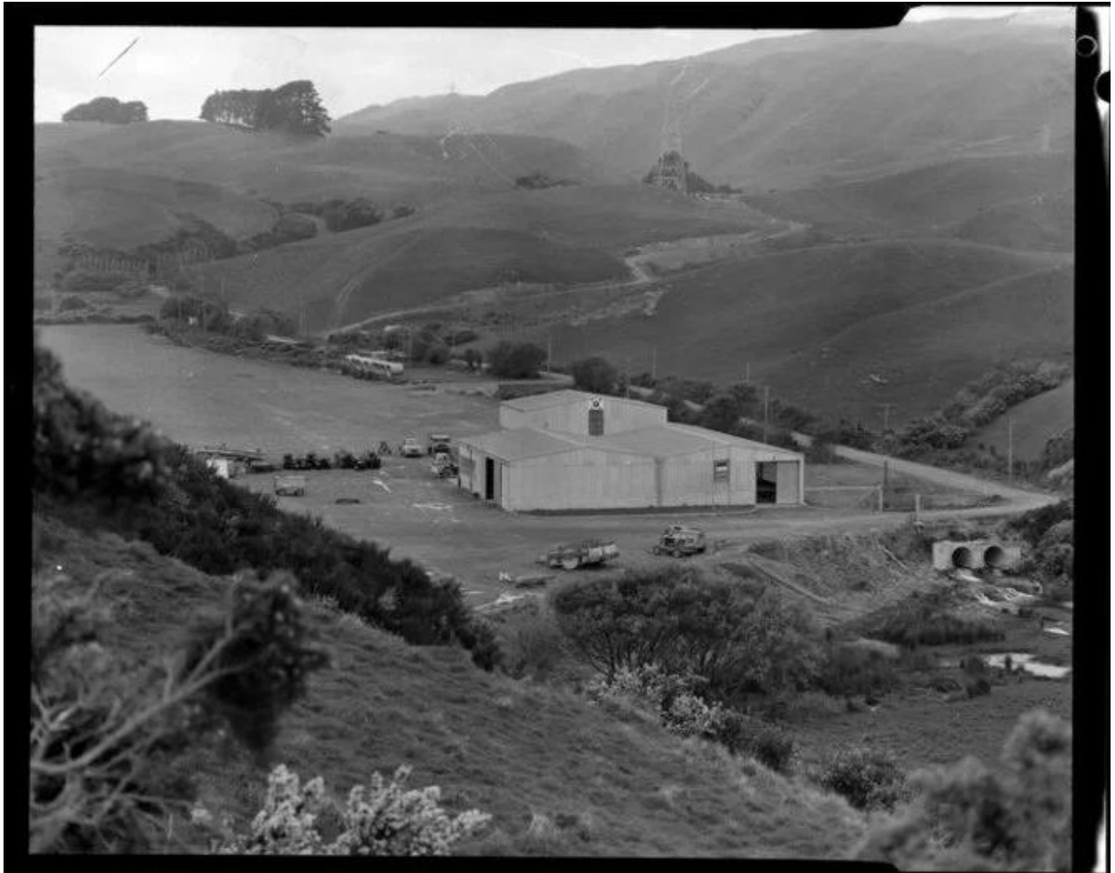
Fletcher Construction Plant at Tawa | Items | National Library of New Zealand | National Library of New Zealand Date 1967 Reference 1/2-215681-F Description Fletcher Construction Plant at Tawa, photographed by K E Niven and Co of Wellington
