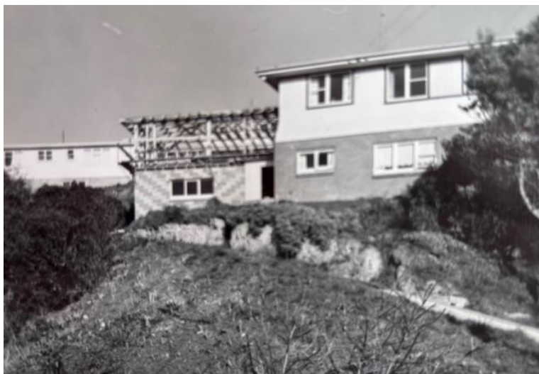
Redwood Ave rumpus room being added
